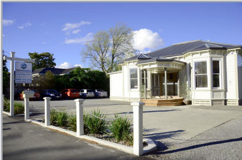
Our new custom built premises in Victoria Street, Masterton
